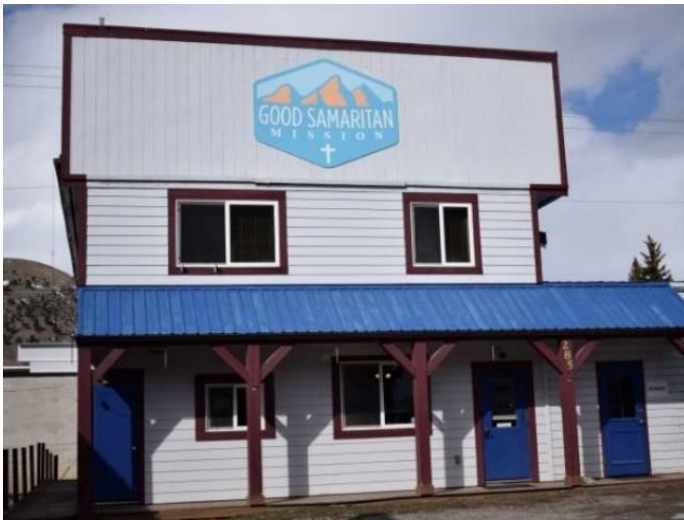
Current Facility Front Entry
